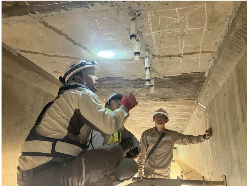
Pilot Bridge Repair Works (Nammone Bridge)
