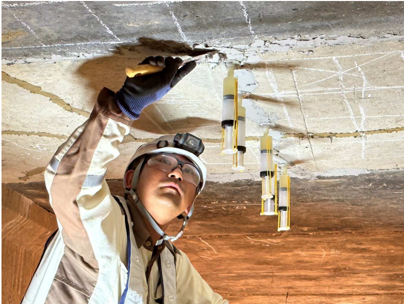
Pilot Bridge Repair Works (Nammone Bridge)
