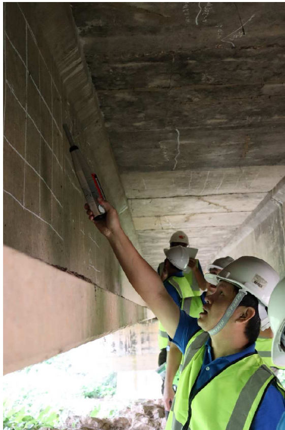
Intensive Bridge Inspection and Repair Training (On-site Training for Pilot Inspection)
