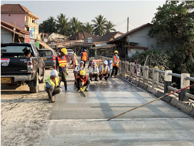
Pilot Bridge Repair Works (Nammone Bridge)
