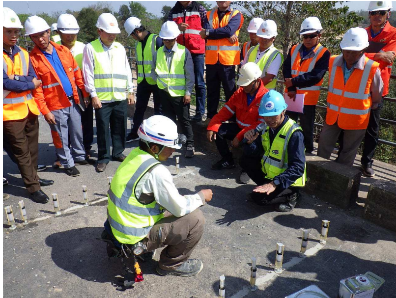
Pilot Bridge Repair Works (Xe Bangnouan Bridge)
