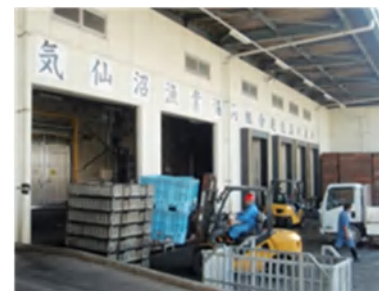
Industrial Freezer Warehouse
